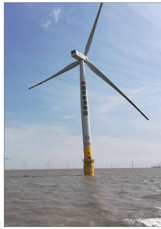
Dongtai Offshore Wind project
